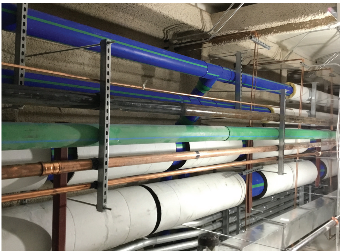
Aquatherm pipe sizes ranging from 3/4-in. to 24-in. installed at the Seminole Hard Rock Hotel & Casino.
