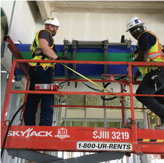
Kirlin's installation team heat-fusing large-diameter Aquatherm pipe using a prototype McElroy Acrobat™ 630 at the Seminole Hard Rock Hotel & Casino.
