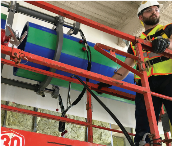
Trying to weld large diameter pipe overhead in tight spaces can be difficult and time-consuming, but the decision to use heat-fused Aquatherm pipe helped keep this project on schedule.
