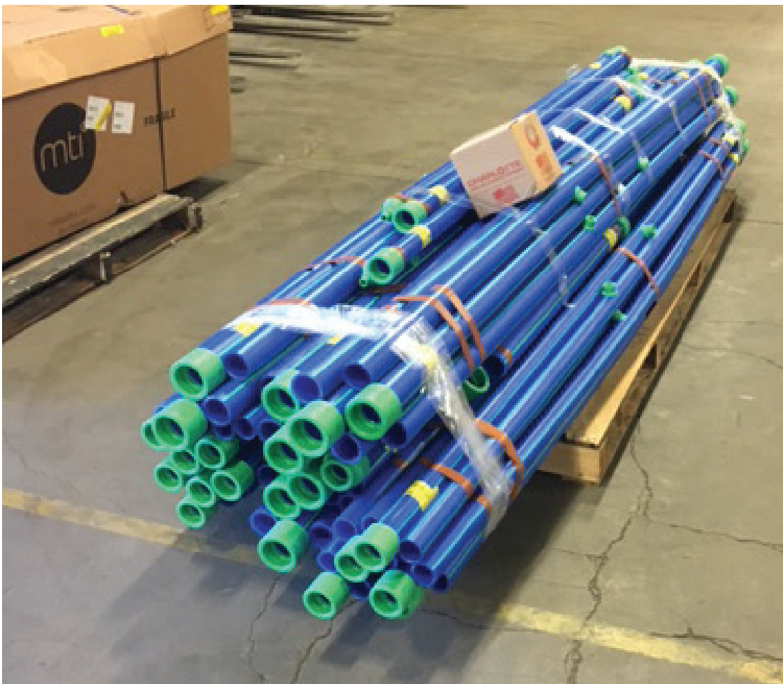
Offsite fabrication helped speed this project along, as ready-to-install risers were shipped directly to the jobsite.
