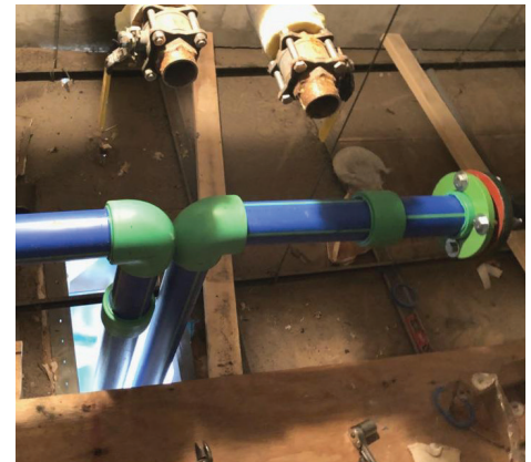
The 22-story Windsor Over Peachtree condominium building features commanding views of downtown Atlanta and the surrounding area (left). Above: Aquatherm pipe in place at Windsor Over Peachtree. Its virtually leak-free performance impressed the installing contractor.
