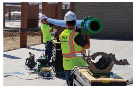
Depending on size and wall thickness, polypropylene pipe can weigh up to 70% less than carbon steel pipe.
