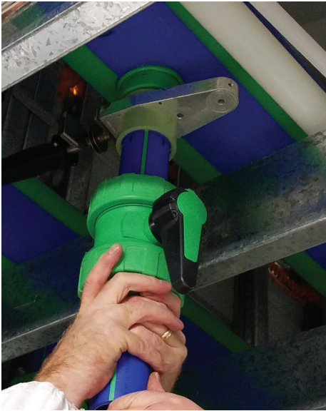
Socket fusion (shown here) is one method of heat-fusing polypropylene pipe and fittings.
