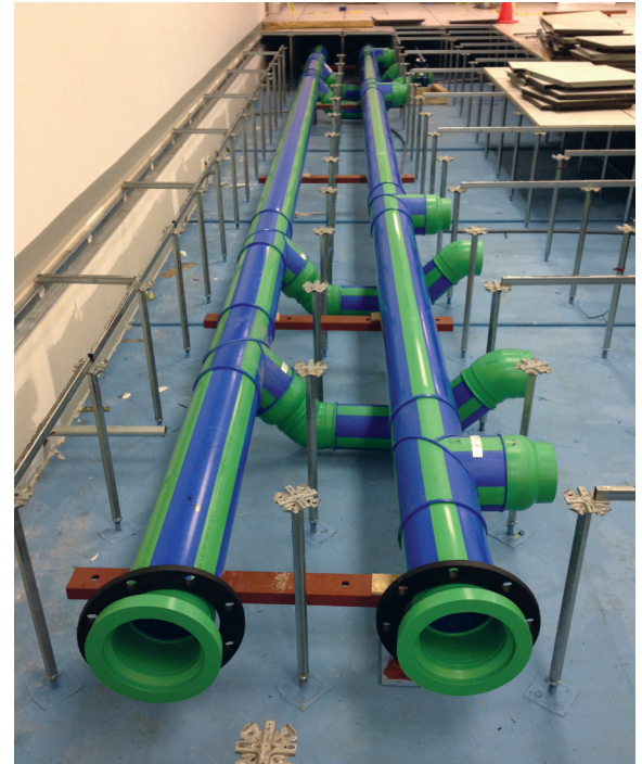
Polypropylene can be fabricated into long, seamless assemblies without welding, gluing, crimping, or introducing VOCs into the data center environment.
