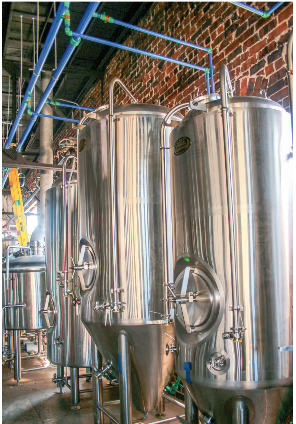
Aquatherm Blue Pipe connects the glycol chiller to the brewery's 16 fermentation and serving tanks.
