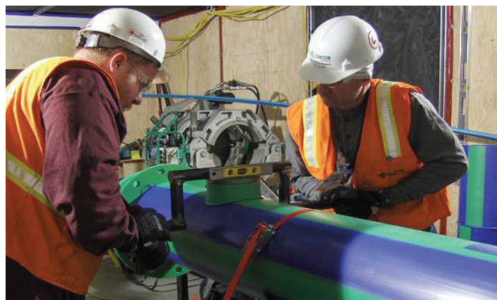
Aquatherm’s clean heat fusion process (below) and long life make it an ideal choice for mission-critical cooling applications such as data centers.
