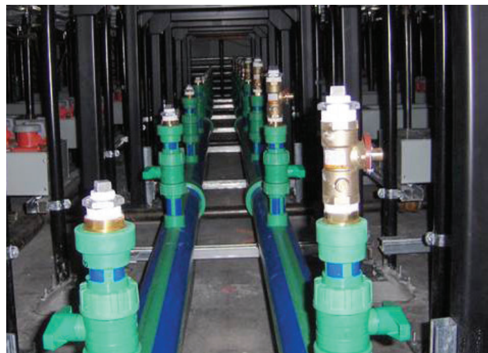
Aquatherm’s clean heat fusion process (below) and long life make it an ideal choice for mission-critical cooling applications such as data centers.
