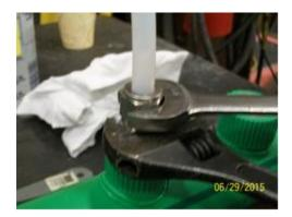
3. Always apply counter torque on the metal portion of the Aquatherm fitting when tightening the connection. If the fitting has a hex head, place your wrench on it; a crescent wrench may be too wide for the hex portion, in which case a plumber's wrench or open-end wrench may be necessary. For fittings without a hex head, use a strap or pipe wrench on the PP-R body of the fitting. Excessive torque on the brass may cause the
