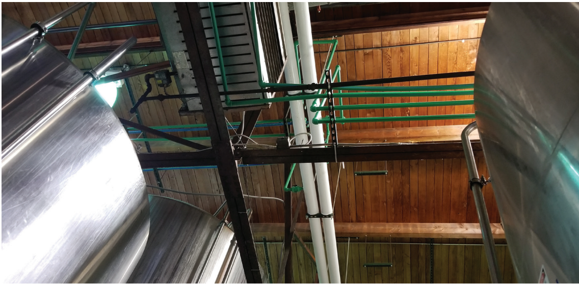
The light weight of Aquatherm pipe made it easy for one person to install, even when working overhead.
