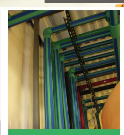
"[Aquatherm is] really a solid product. We haven't had any leaks or other concerns, and we haven't had any issues with the pipe regarding vibration and hammering with the air-operated diaphragm pumps."
