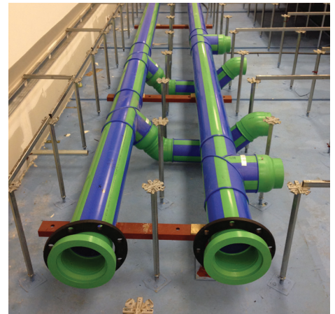
Aquatherm pipe in place during the 2014 renovation of a 1983 building into a modern data center.
