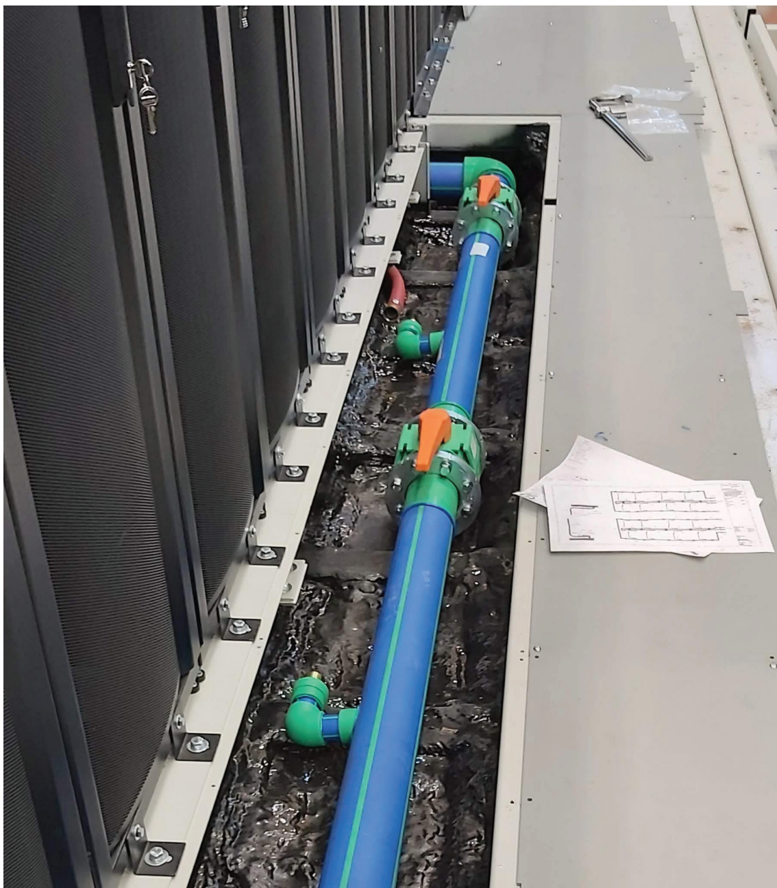
Aquatherm pipe provides a lightweight, durable solution for the self-contained cooling system in a modular data center.
