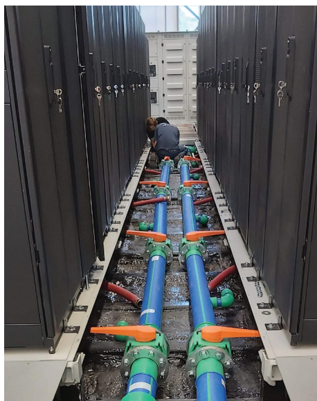
Aquatherm pipe installed (right) in a modular data center and fabricated spools in place and awaiting installation (left).
