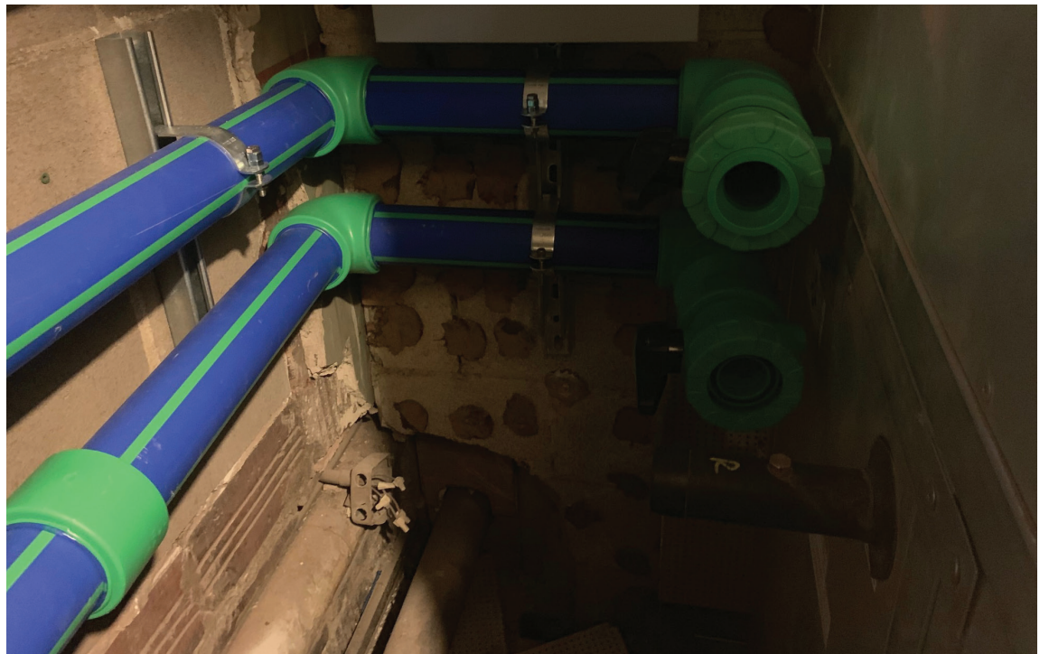
Brand-new Aquatherm pipe in place in the nearly 100-year-old chases at the New South Federal Savings Building.
