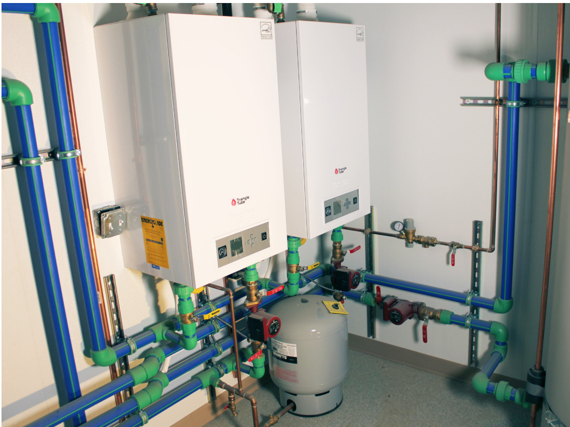
The pods can be utilized for any type of mechanical system, but hydronic systems generally provide the greatest benefit because they involve the most labor.
