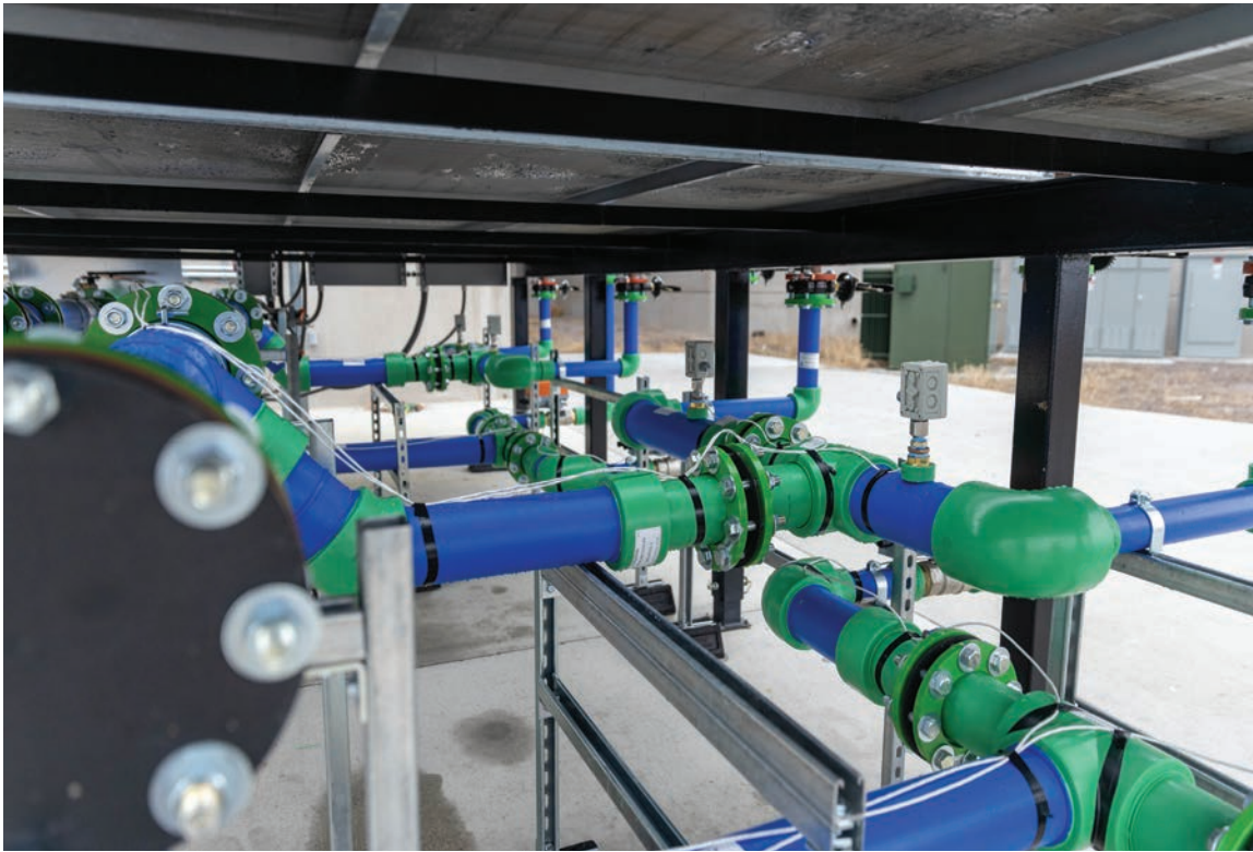
Novva's dry cooler eliminates the need to use mechanical cooling in the colder months.
